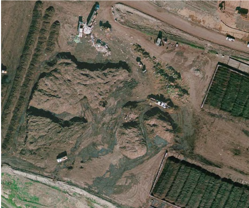
Figure 1-5. Newby Island Landfill Green Waste Facility
