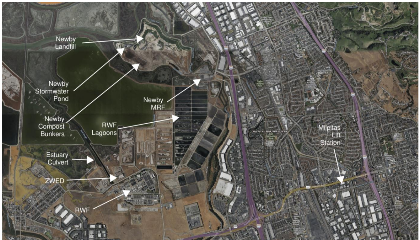
Figure ES-1. Key Odor-Emitting Facilities, Sources, and Surrounding Communities
