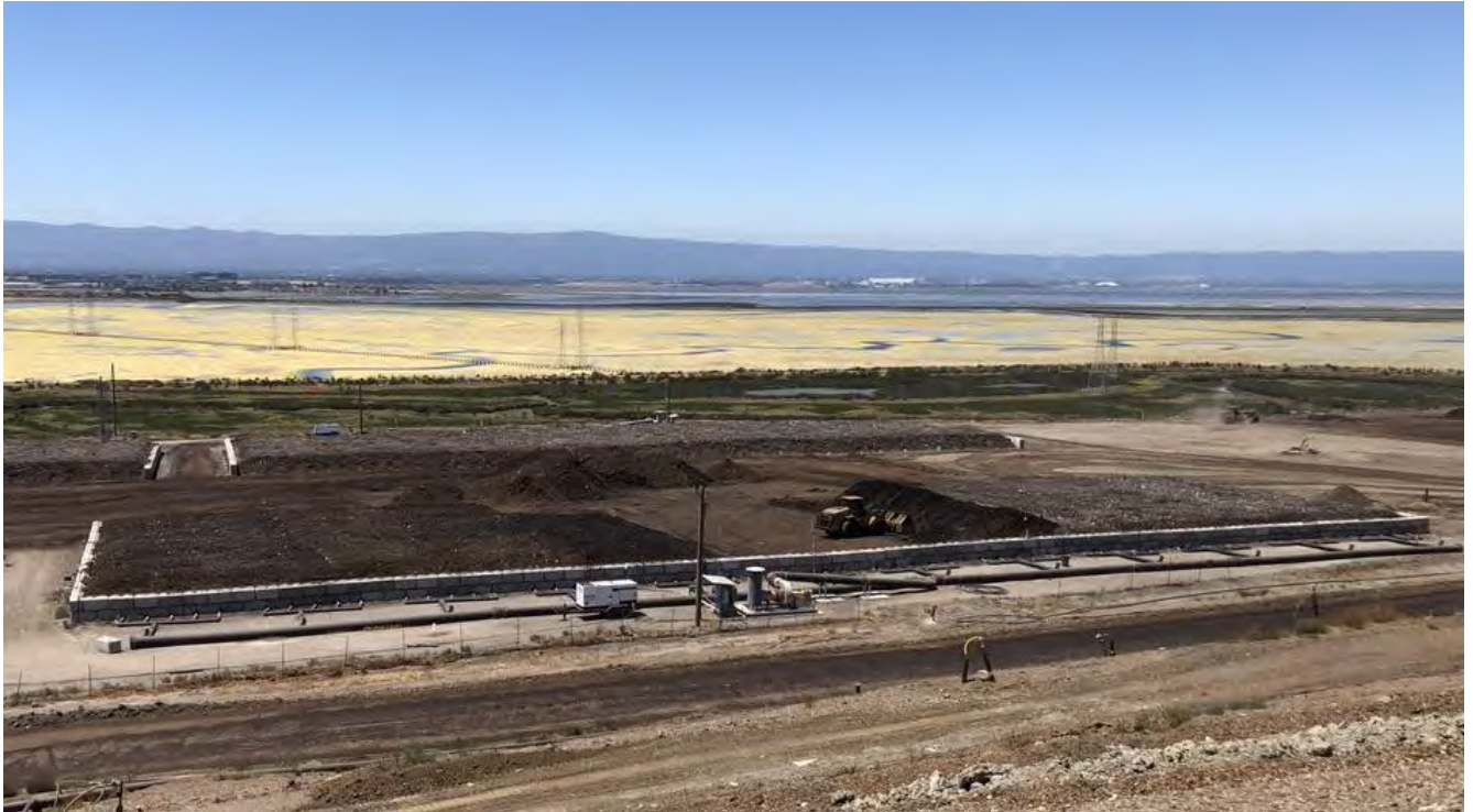
Figure 1-6. Newby Island Landfill Composting Process
