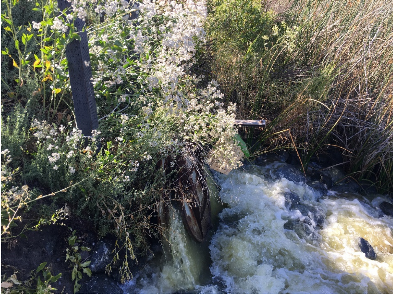
Figure E-12. Bay estuary culvert
