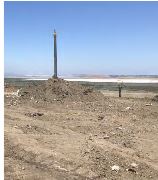
Figure 1-7. Landfill Gas Header
