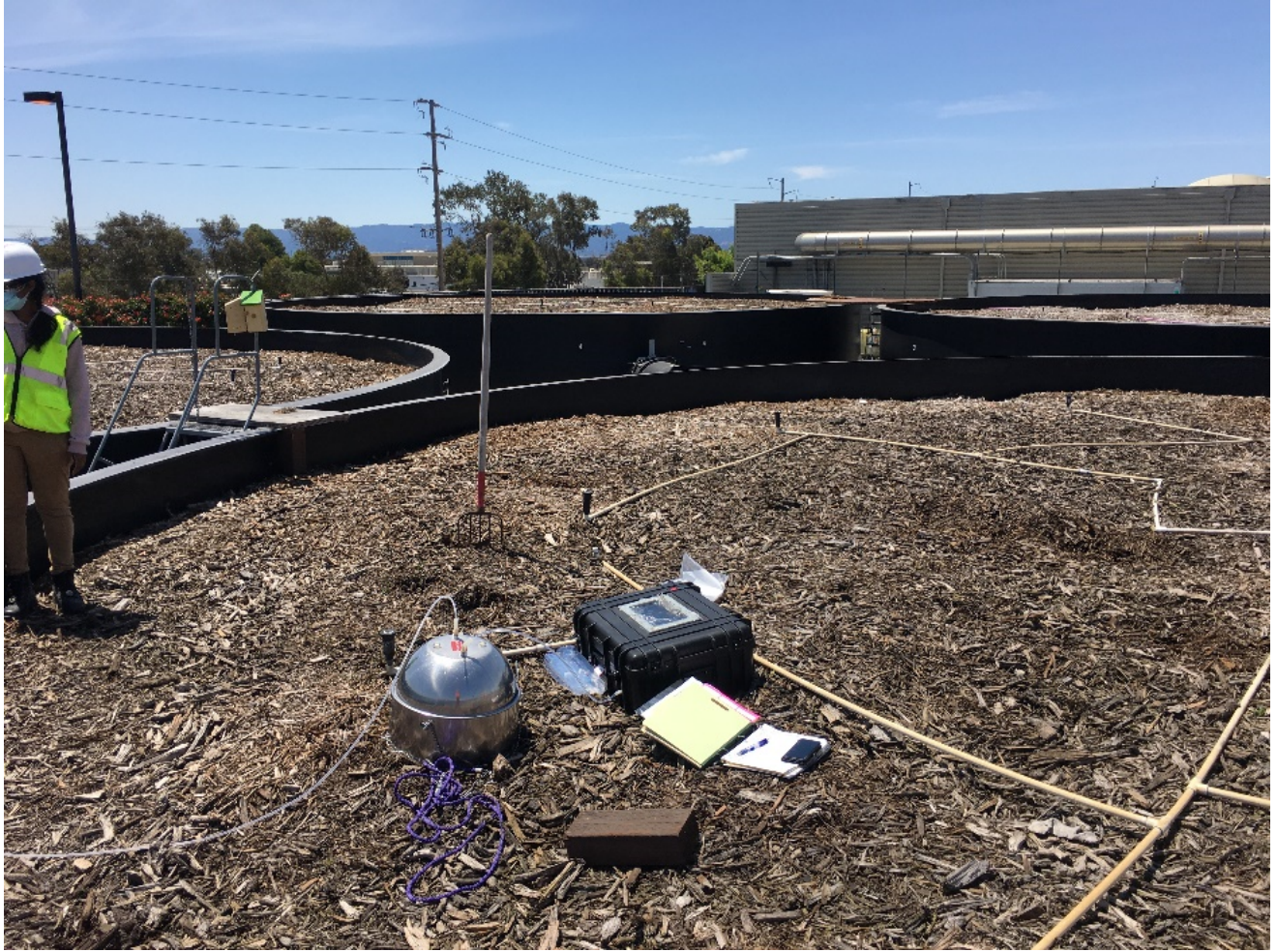
Figure E-13. Vacuum chamber with flux chamber on surface of ZWED biofilter
