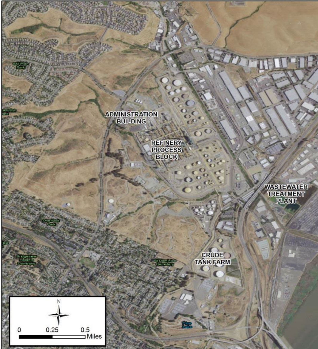
Figure 4. Layout of the Valero Benicia Refinery (Source of information: Valero Improvement Project Environmental Impact Report, June 2008).
