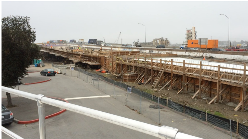
Figure 9: Laney College site, looking southeast along I-880
